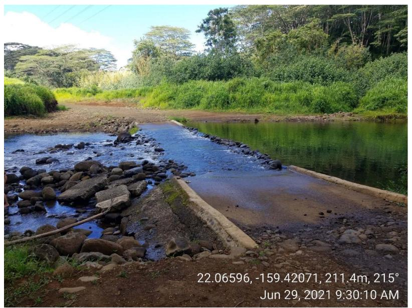
**Figure 9: Photograph of the damaged Queensland Crossing** Note the recently constructed boulder alignments connecting the concrete remnants of the original crossing.
